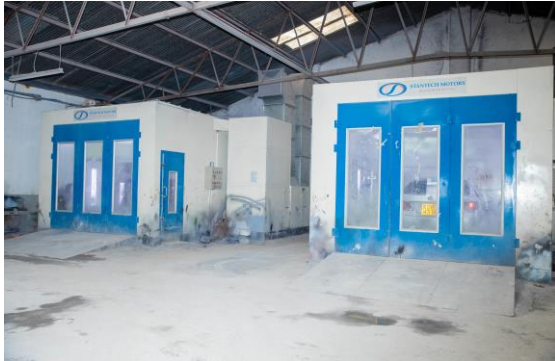
State of the Art Modern Spray Booth
